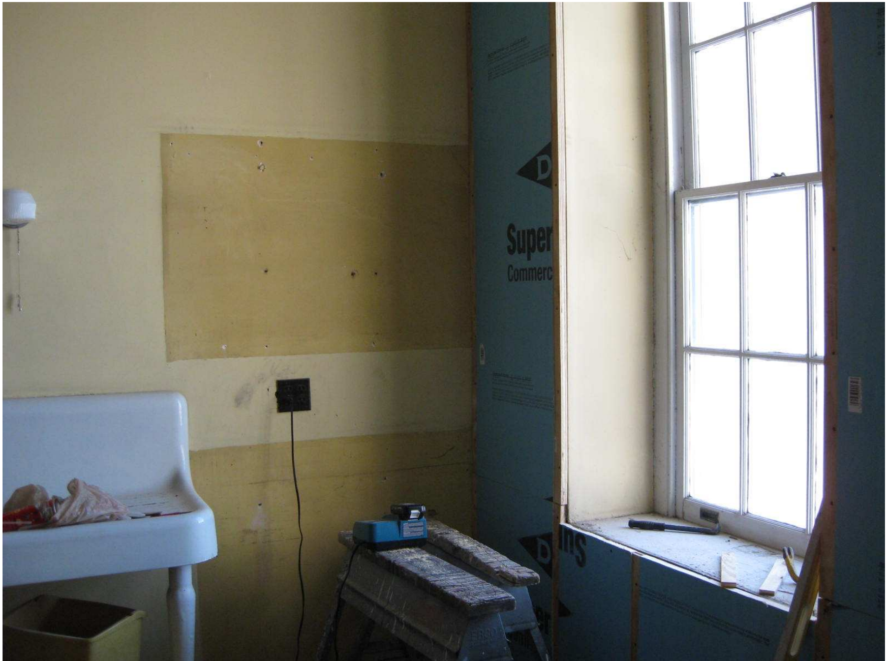
The Outside Wall is Insulated (Last Peek at the Old Sink) – 7/19/09
