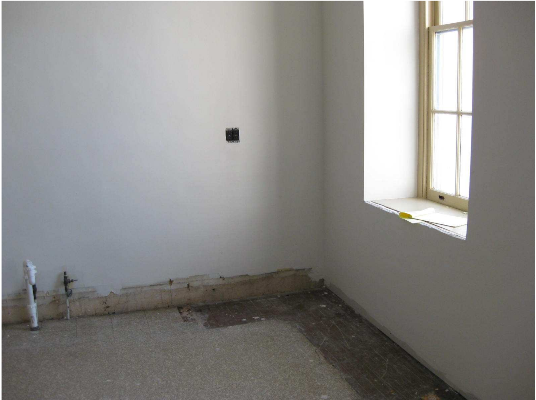
New Paint (The Old Sink is Gone) – 8/16/09
