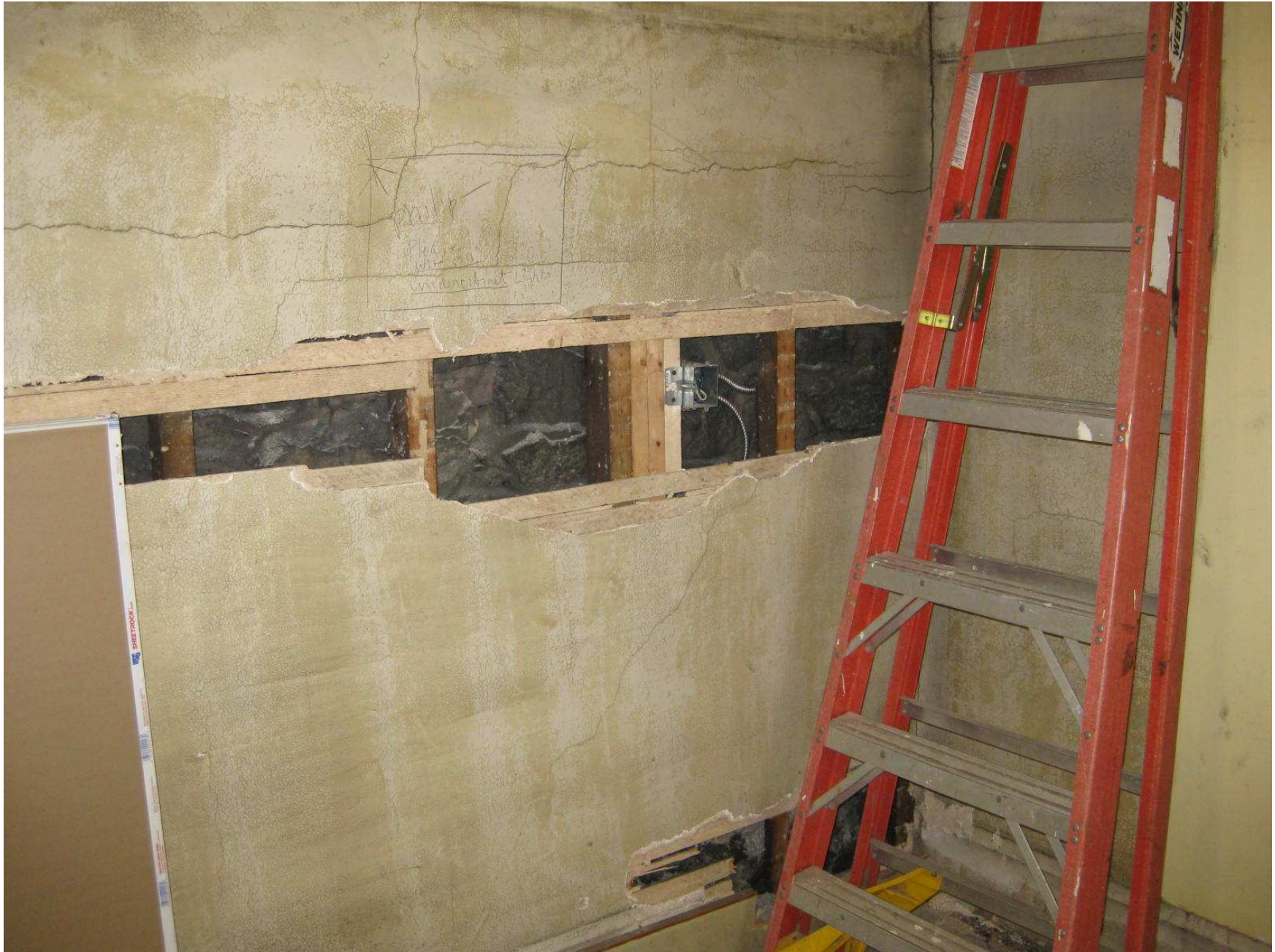
The Wiring Goes In – 7/19/09
